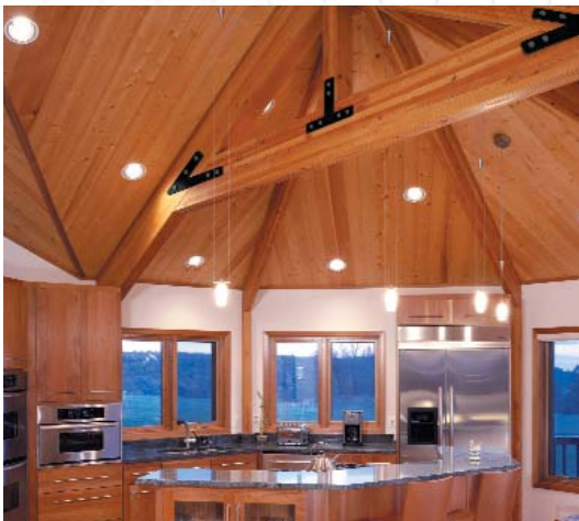
A collection of pre-finished connectors for exposed timber construction, the Architectural Products Group, combines structural integrity with decorative architectural detailing to offer increased design flexibility. The textured black powder-coat finish offers an attractive product that is meant to be seen.
